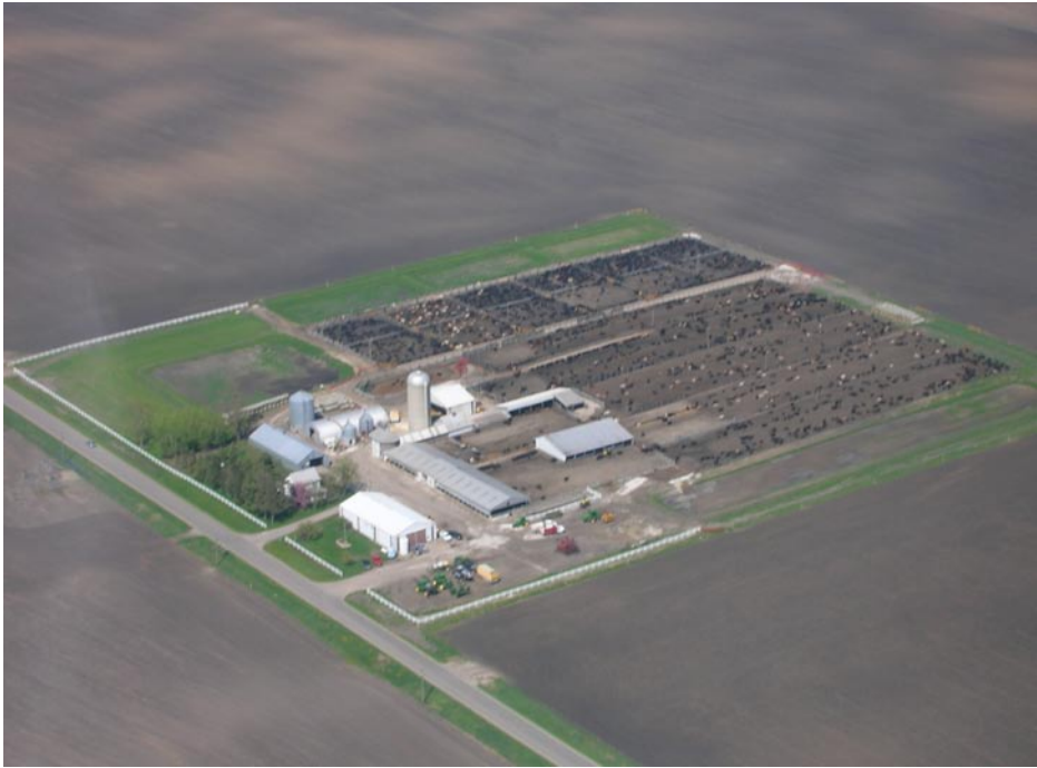
Completed Project: After construction and during vegetation establishment with 2600 head of cattle
