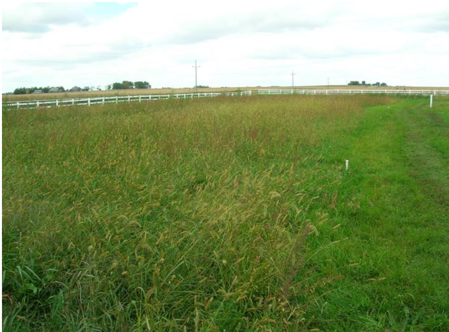
Completed Vegetative Treatment Area
