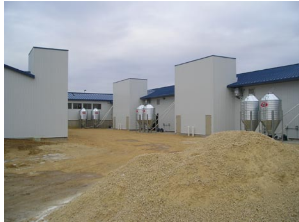
View from Back Side of Buildings
