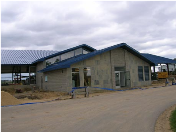
Front during Construction
