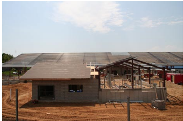
Parlor under Construction
