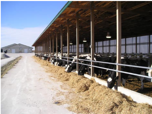
Open Front Heifer Building
