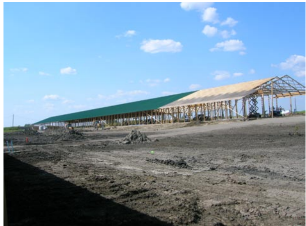
Free Stall Barn Under Construction
