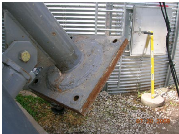
Base plate of tower leg.
