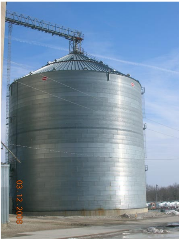
Bin with rusted interior.
