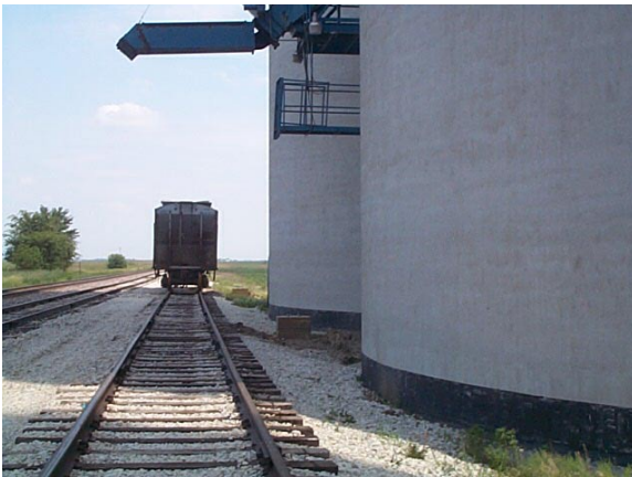
New Rail Load Out location
