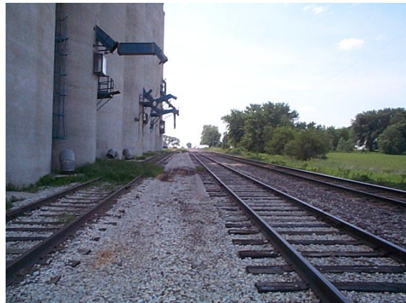
New Rail Load Out location
