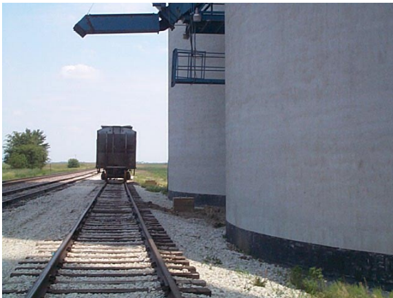
New Rail Load Out location
