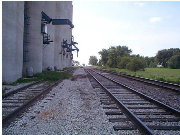
New Rail Load Out location
