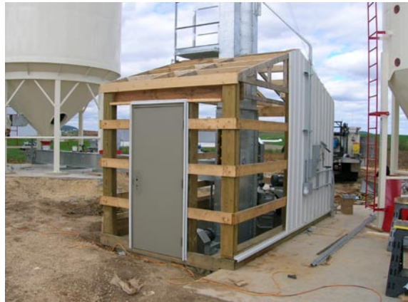
New Boot Pit enclosure
