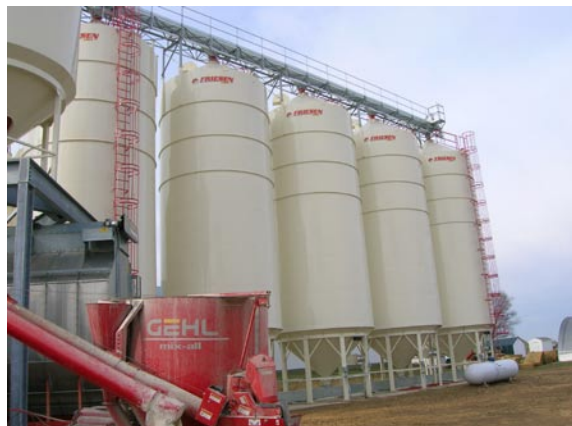
Storage Bins with Aeration
