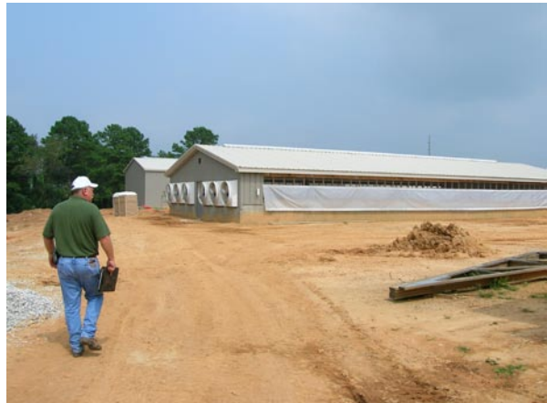
Exterior of Breeding/Gestation Building
