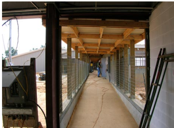
View down Covered Walkway between Buildings
